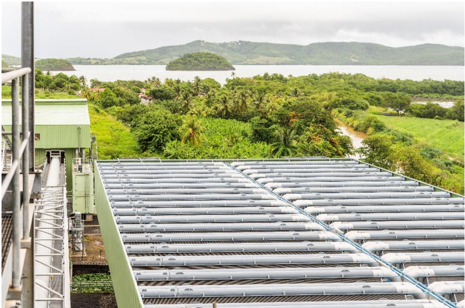
Installation de la centrale Galion 2 © Albioma
